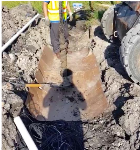
Figure 3.9 Drilling the first borehole with a skid-steer auger.
