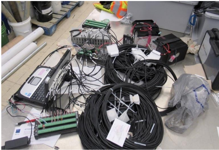
Figure 3.4 Laboratory practice wiring.
