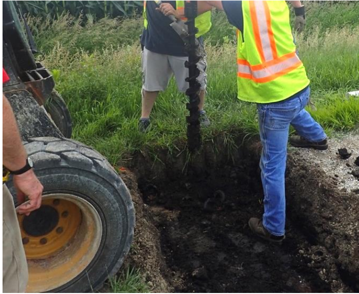
Figure 3.9 Drilling the first borehole with a skid-steer auger.
