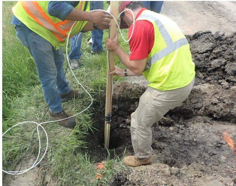
Figure 3.11 Installation trial with the developed installation tool for GS1.
