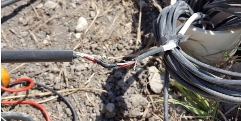
Figure 5.1 Cable splicing for the short cables.
